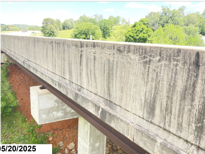
Span 2, left. Parapet wall horizontal cracking.
