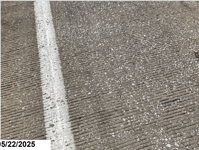
Spans 1 - 3: Transverse and longitudinal cracking.
