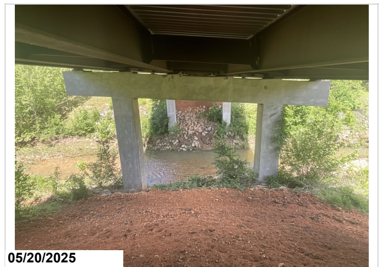
Typical intermediate bent.
