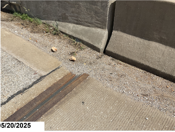
Abutment 1 & 2, Gutter Lines: Debris impact. 12LF CS2
