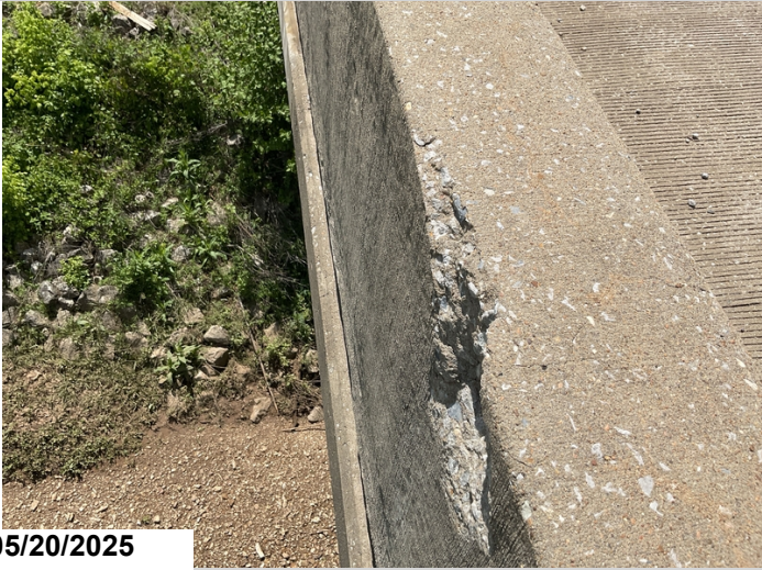
Span 2, Right: Spalling. 1LF CS3
