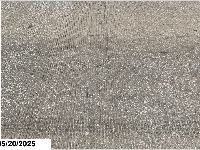
Span 2: Cracking. 564SF CS2
