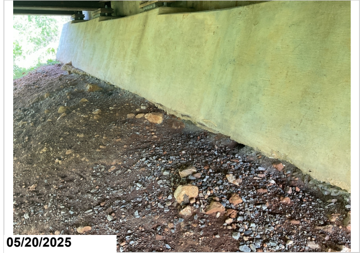
Abutment 2: Minor erosion.
