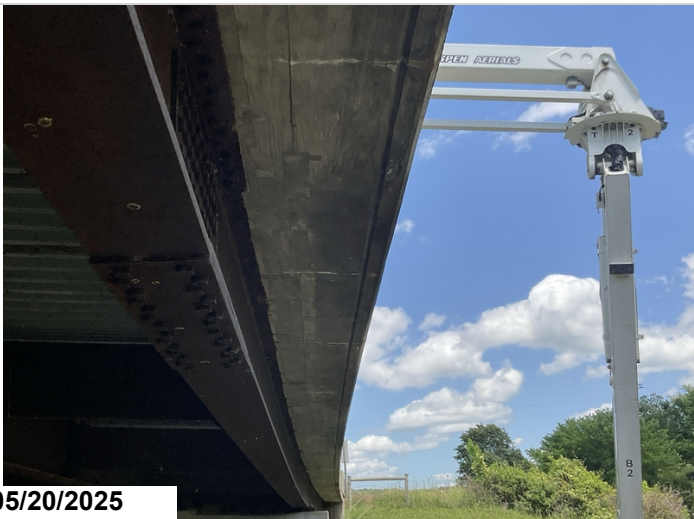
Spans 1 - 3, Right, Overhang: Cracking with efflorescence with build up. 30SF CS3
