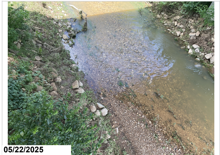
Areas of displaced rock in the channel beneath structure.
