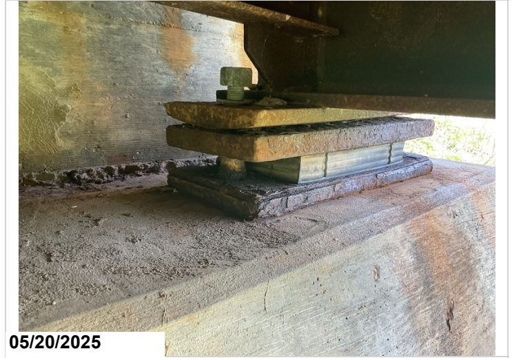
Abutments 1 & 2, Girders 1 - 6: Active corrosion with flaking rust.
