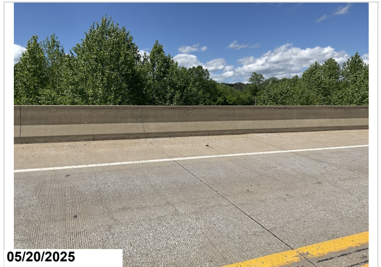
Span 1 - 3, Left & Right: Cracking. 234LF CS2
