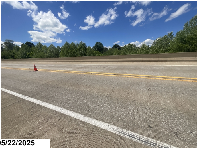
Spans 1 - 3: Abrasion in the wheel paths. 1160SF CS2
