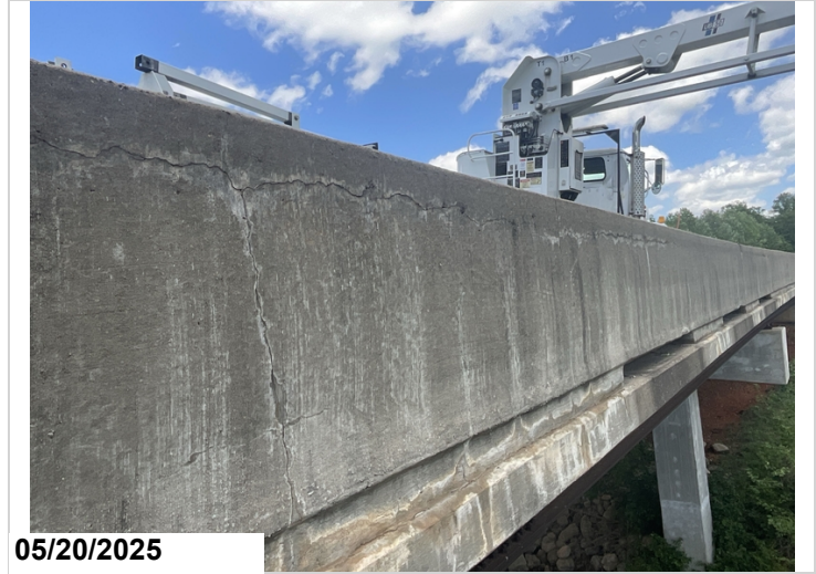
Span 2, right. Parapet wall cracking.
