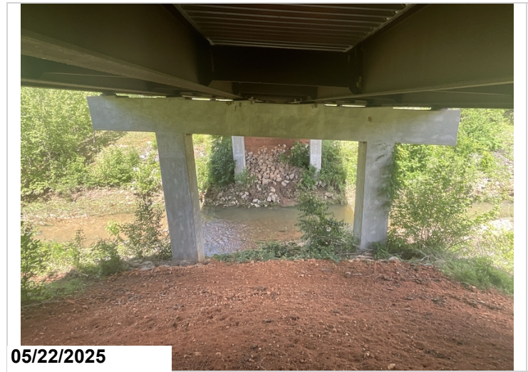
Typical intermediate bent.
