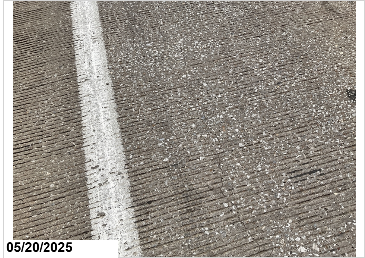
Span 1: Cracking. 280SF CS2
