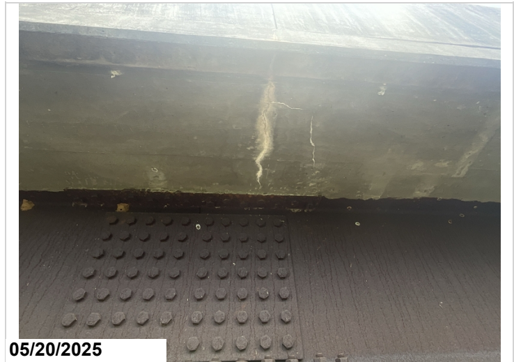
Spans 1 - 3, Left, Overhang: Cracking with efflorescence with build up. 44SF CS3
