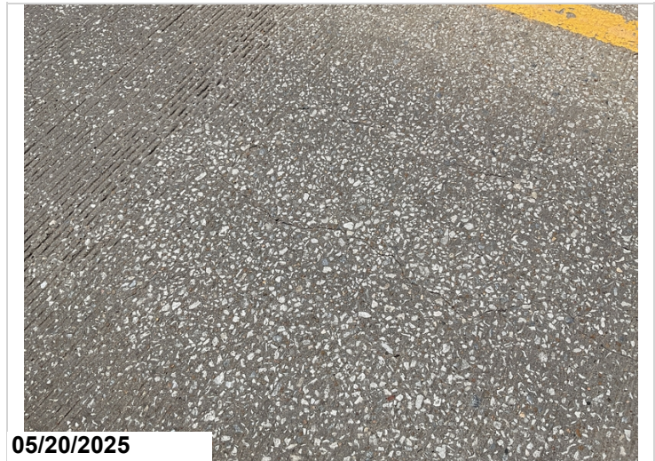
Span 3: Cracking. 412SF CS2
