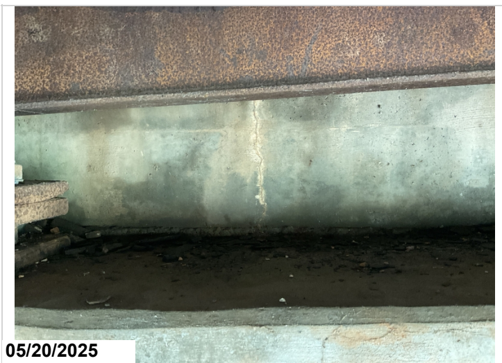
Abutment 1 & 2: Cracking with efflorescence. 3LF CS2
