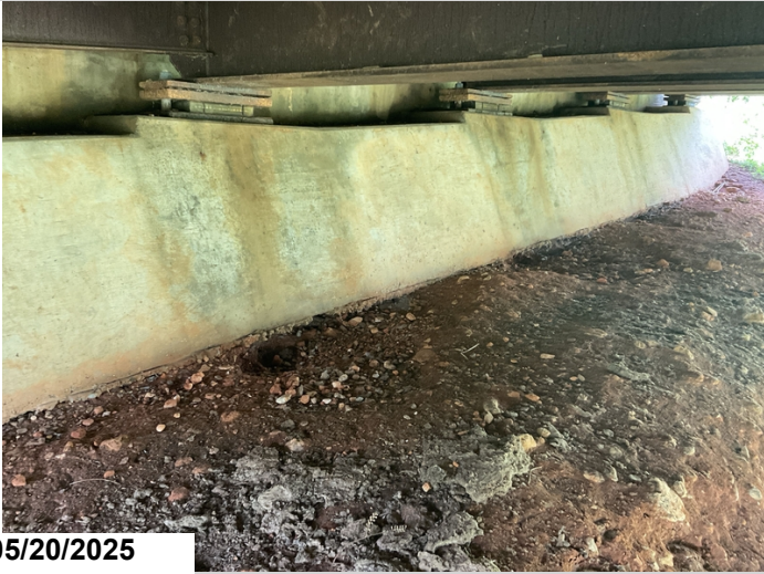
Abutment 1: Minor erosion.
